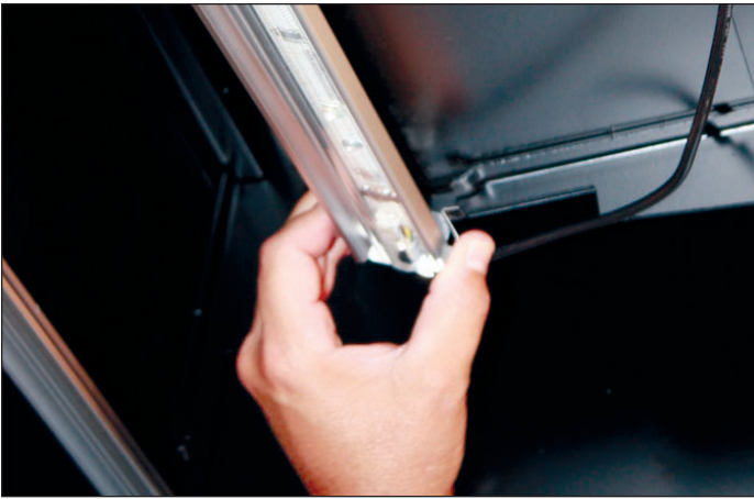
Fig. 19 Remove the old LED luminaire
