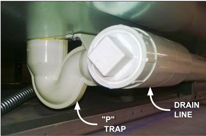
Fig. 11 "P" trap; drain line
