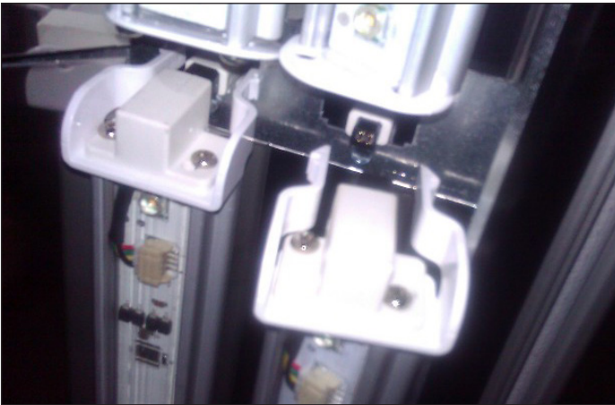
Fig. 20 Squeeze the latching clips and pull the luminaire free
