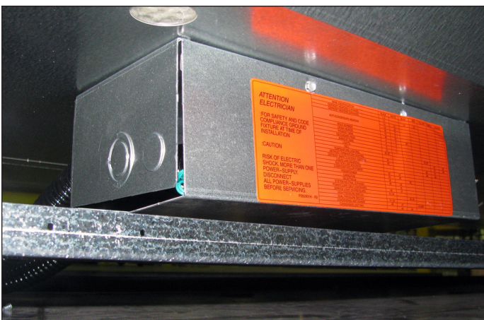
Fig. 12 Junction box beneath case
